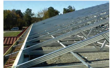
With the assistance of the precise layout, connection, and engineered bracing diagrams (an Ultra-Span system exclusive!) that **All-Span** provided, the truss installer was able to retrofit the Ennis school in just two weeks! And, by working evenings and weekends, no class time was lost (great news for the parents and educators, bad news for the kids!)
