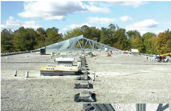
Adequate installation and maintenance access for the new rooftop units was easily accomplished by designing and building a large mechanical "room" into the trusses covering those areas where the units would be located.
