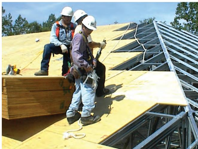
*The STABILIZER® not only spaces trusses and braces, but can remain in place as roof sheathing is applied. This is just one more way to save money on your project.*
