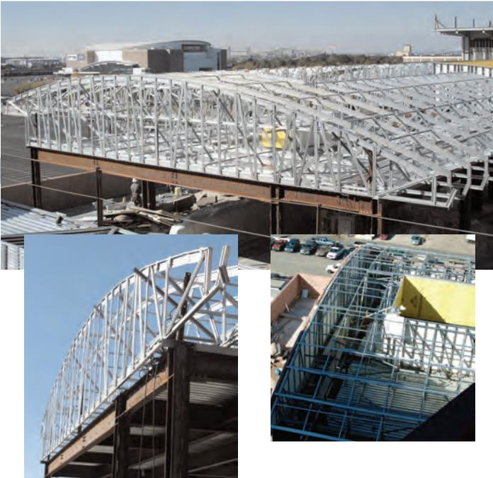
This truss profile employs both a radius top, and built-in gutter detail.
